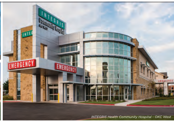
INTEGRIS Health Community Hospital - OKC West
