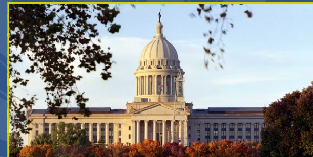
Oklahoma State Capitol Exterior Rehabilitation
